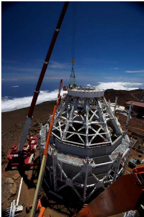
Fig. 9 Progress of site construction as of August 2014 showing the installation of the head ring on top of the pier cone [20].
