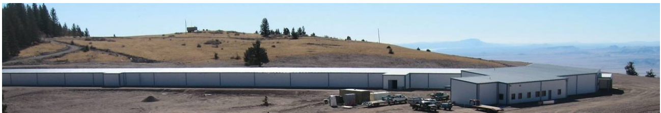
Figure 3. The beam combining and delay line facilities for MROI. Note the 200m long portion of the building extending off to the left in this picture, which houses the delay lines. Light beams enter the building from the center of the array arms on the right side of the photograph.
