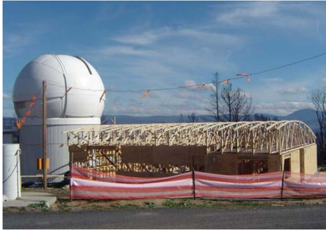
Fig 6. Laser and Control Room Construction
