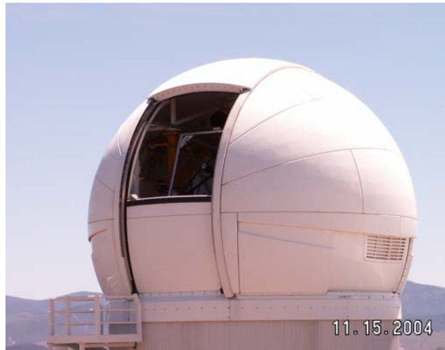
Fig 16. BDS in IceStorm enclosure
