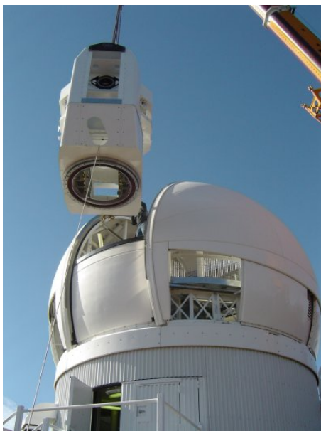
Fig 8. Installation of the 1.8m telescope
